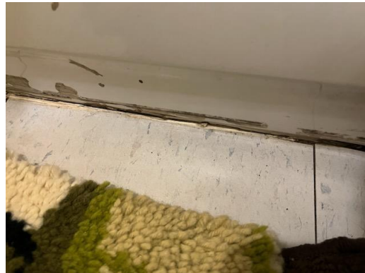
1912-4 12"x12" Floor Tile/Adhesive Interior Bathroom/Family Room
